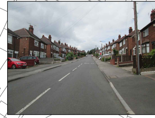
View up Prospect Road towards Hillview Road
